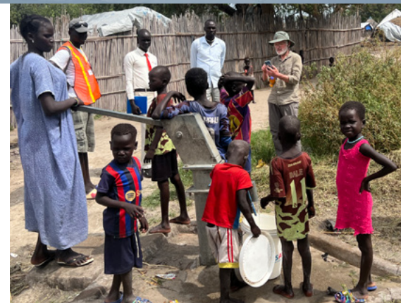
Diel #1 water well. One of 67 wells completed so far by AHPSS.
