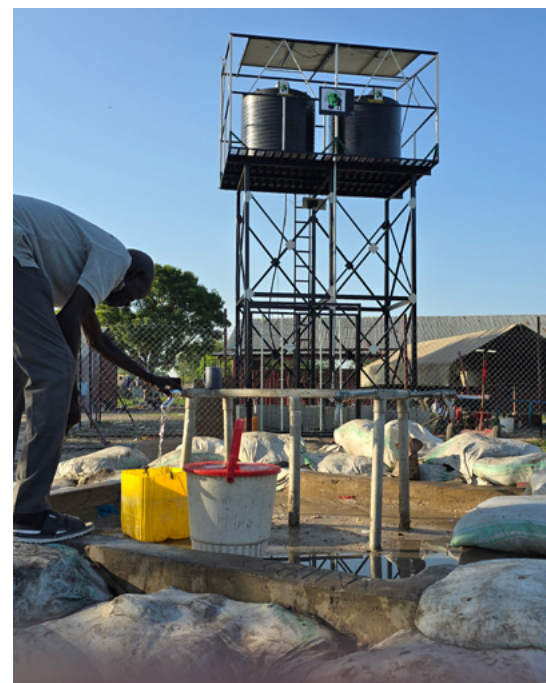
Water yard for elementary school students at Old Fangak.
